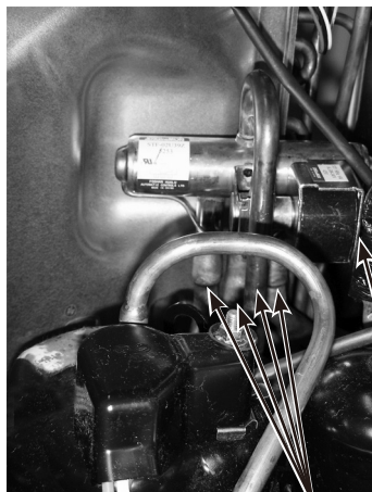
Brazed parts of 4-way valve
